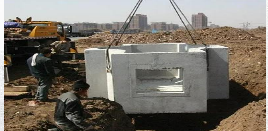
Cable well installation site
